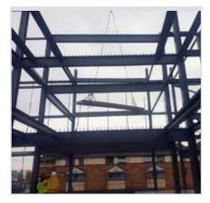
Care must be taken during the lowering of precast planks through steelwork. Tag lines to be used to guide the units through the steel.
