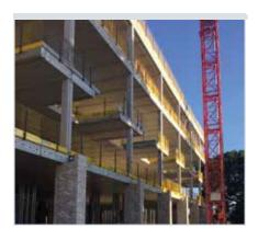
All open edges will have a propriety edge protection system or scaffolding erected to provide edge protection.
