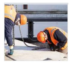
The slinging of the units will only be carried out by a trained CPCS trained slinger/banksman. The slinger will ensure that the load is secure and safety chains are fitted to the precast floor units correctly prior to carrying out the lift. Safety chains are attached at low level. The slinger/banksmen are to ensure safe foot placement when on the back of the trailer attaching lifters
