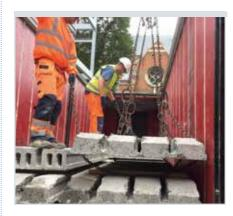
All chains and lifting equipment will be visually inspected and recorded on a LOLER check sheet. This document will be completed weekly. Chains will have a visual inspection each time they are used, checking for damage from buckling or frayed slings. If the chains or slings are damaged they are discarded and marked -
